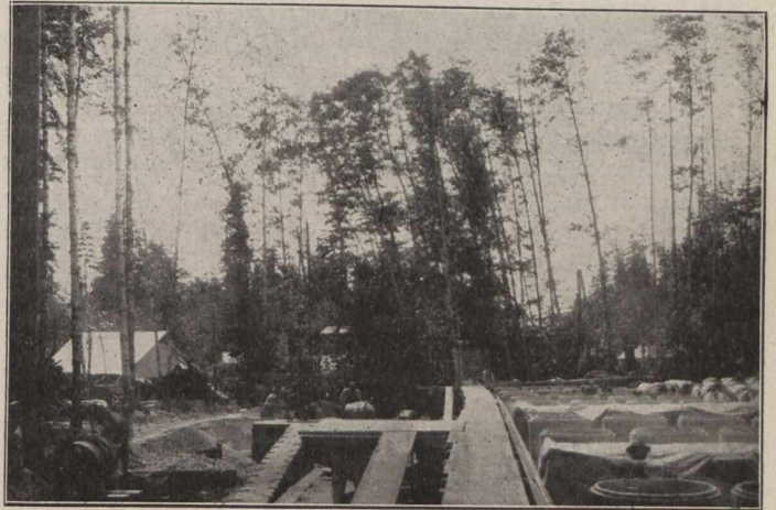
Fig. 8.—Site of Manufacture of Pipe Sections at Cooper's Cove.
