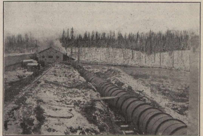
Sandy Falls Power Development—New Steel Pipe Leading to Power House.
