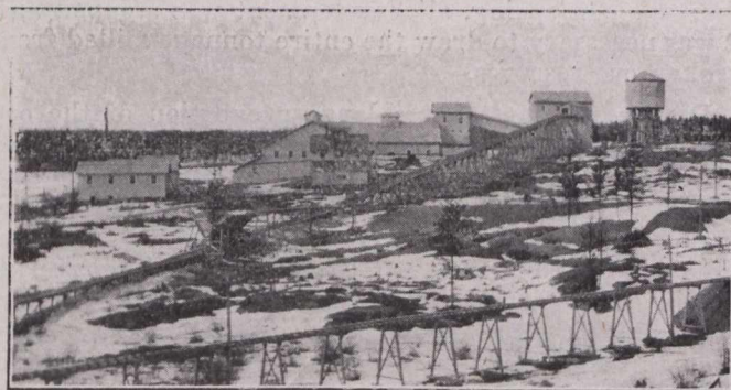
Tough-Oakes mill and cyanide plant, Kirkland Lake. □
