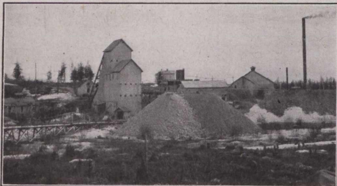
Shaft-house and compressor house, Tough-Oakes mine.
