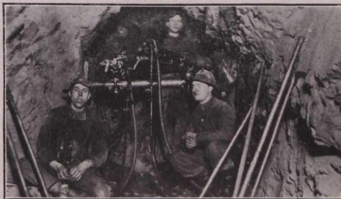
Drifting with Leyner-Ingersoll machine, Tough-Oakes mine, Kirkland Lake.
