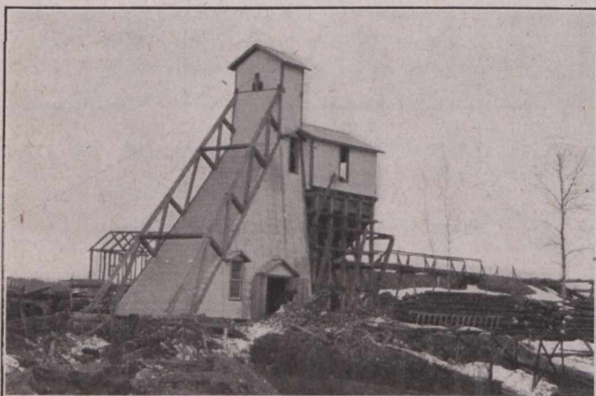
New shaft-house at Teck-Hughes mine, Kirkland Lake.
