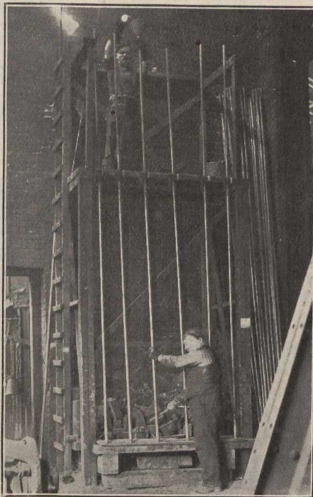
Fig. 2. Filling the Tubes with Sand.
