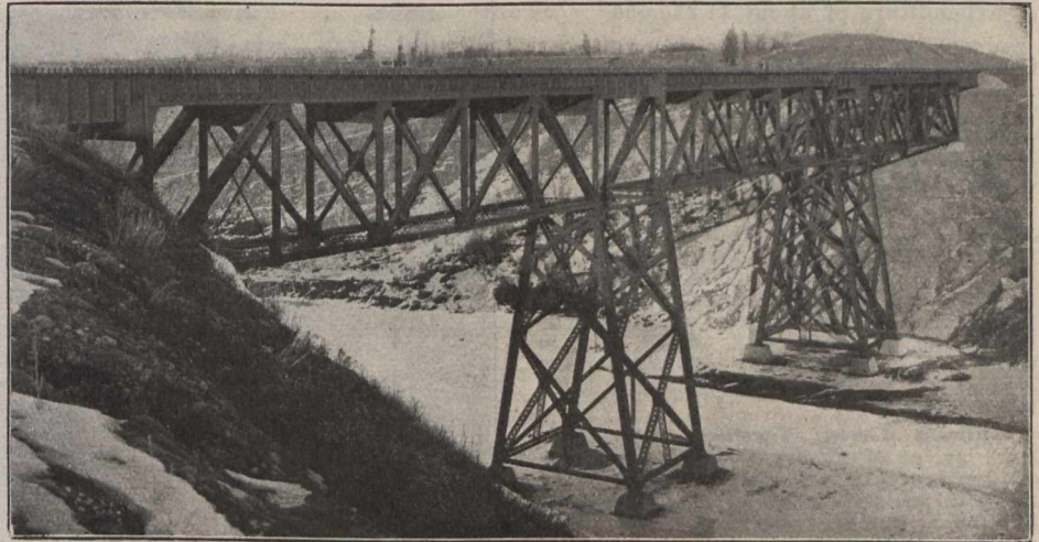
The Grand Trunk Pacific Railway Wolfe Creek Bridge.
