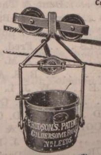
61—Rope Bucket, with R. H.'s Patent Catch for Wire Rope
