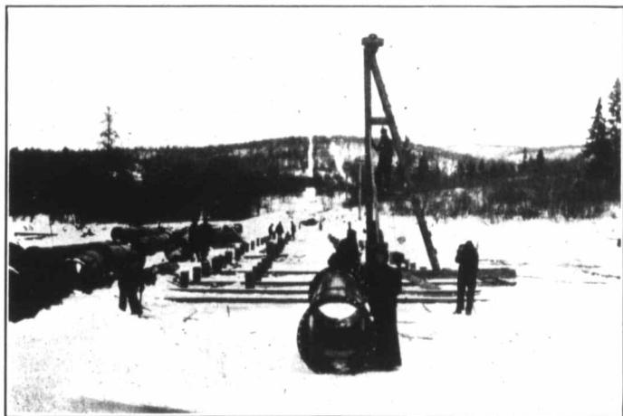
Driving Cofferdam Piles for Intake Pipe. Tunnel Survey Line showing over the Hill.
