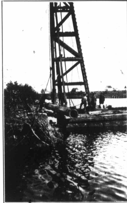
River Pipe in Slings, ready to cast off from Bank.
