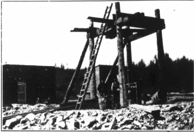
Sinking Shaft by Hand Labour. Head Gear and Winch in course of Erection.
