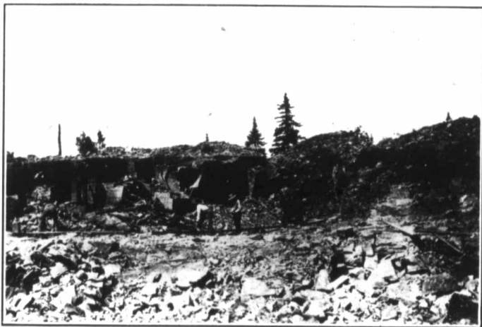
Excavating for Reservoir.
