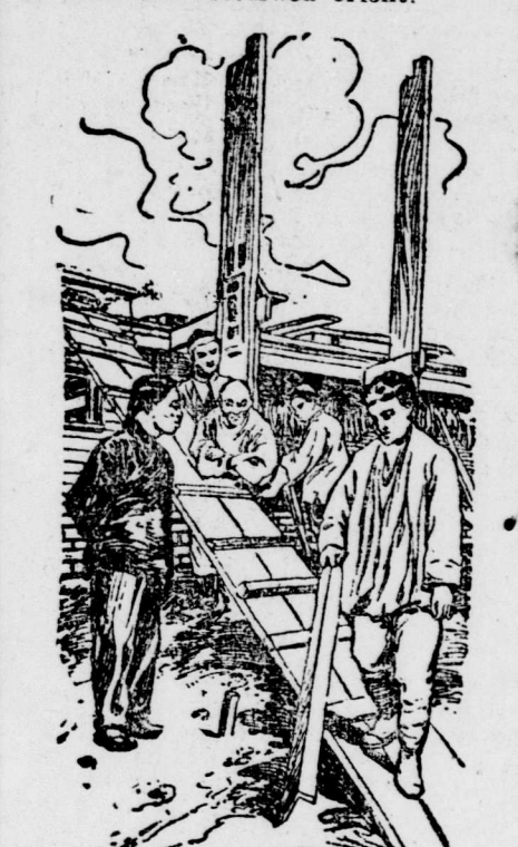
MANCHURIAN LABORERS BUILDING RUSSIAN BARRACKS.
