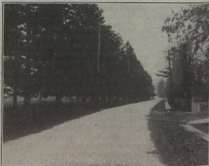
Quebec-St. Augustine Highway, hot-mix asphalt, now under construction. Laid on old macadam
