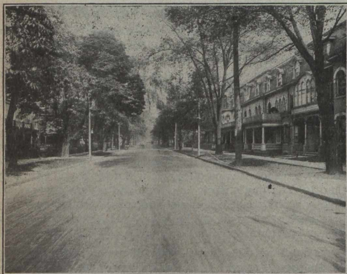
Jarvis Street, Toronto, hot-mix asphalt, surfaced 1901, photo 1917. Repairs negligible
