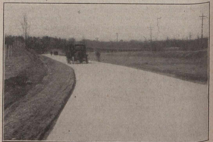
The Construction of Concrete Roads Brings New Business to the Truck Salesmen
