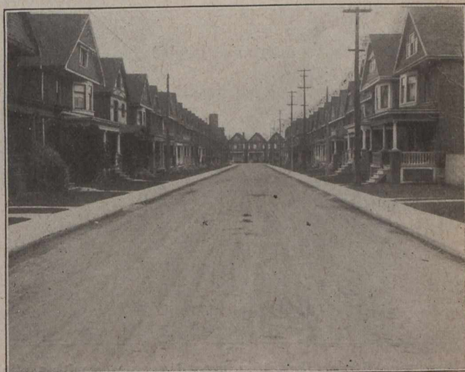
Holton Avenue, Hamilton, asphalt road oil on waterbound macadam. Photo at end of season, 1917
