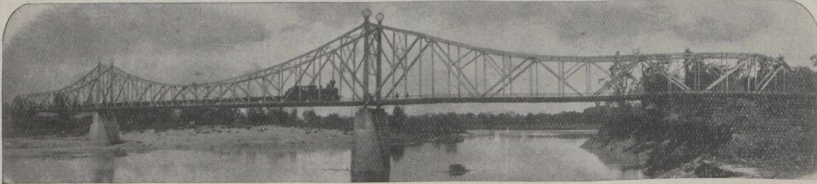
Bridge over the River Menam designed and constructed for the Royal Siamese State Railways.
