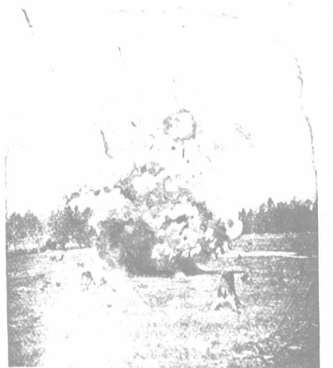
Wheel sharpened to the stump by using Stumping Powder.
