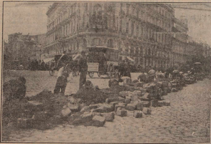
Laying Callender Mains at MADRID.
