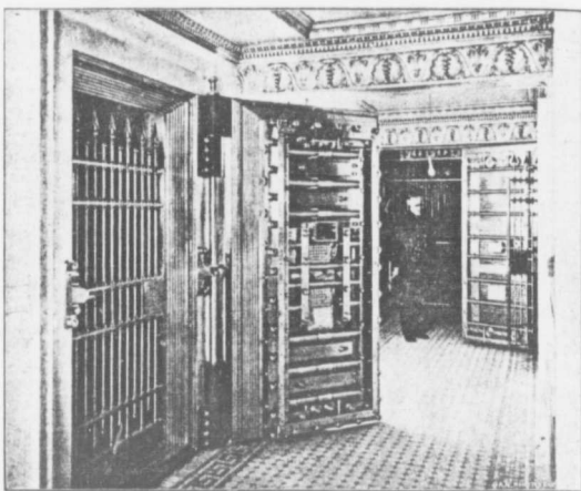
The six ton time lock vault door of
