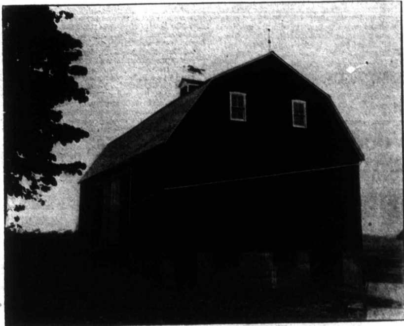
BARN OF WM. PATTON, SOUTH CAYUGA, ONT. Size of Basement Walls, 36 x 60 x 9 feet. Built with Thorold Cement.
