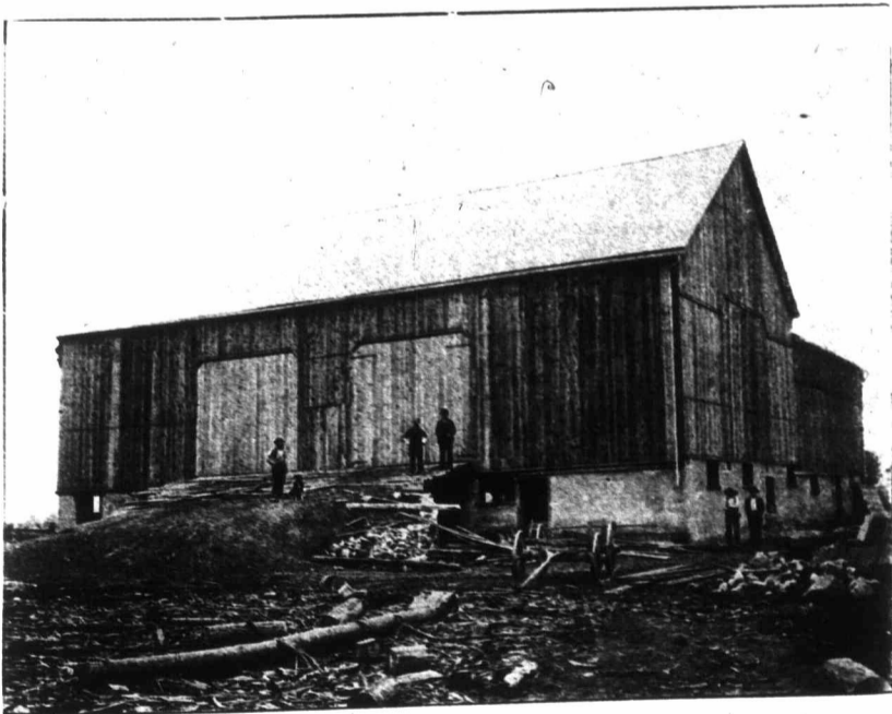
BARN OF ALLAN McMANE, ELMA TOWNSHIP. Basement Walls, 84 x 100 x 9 feet high. Built with Thorold Cement.
