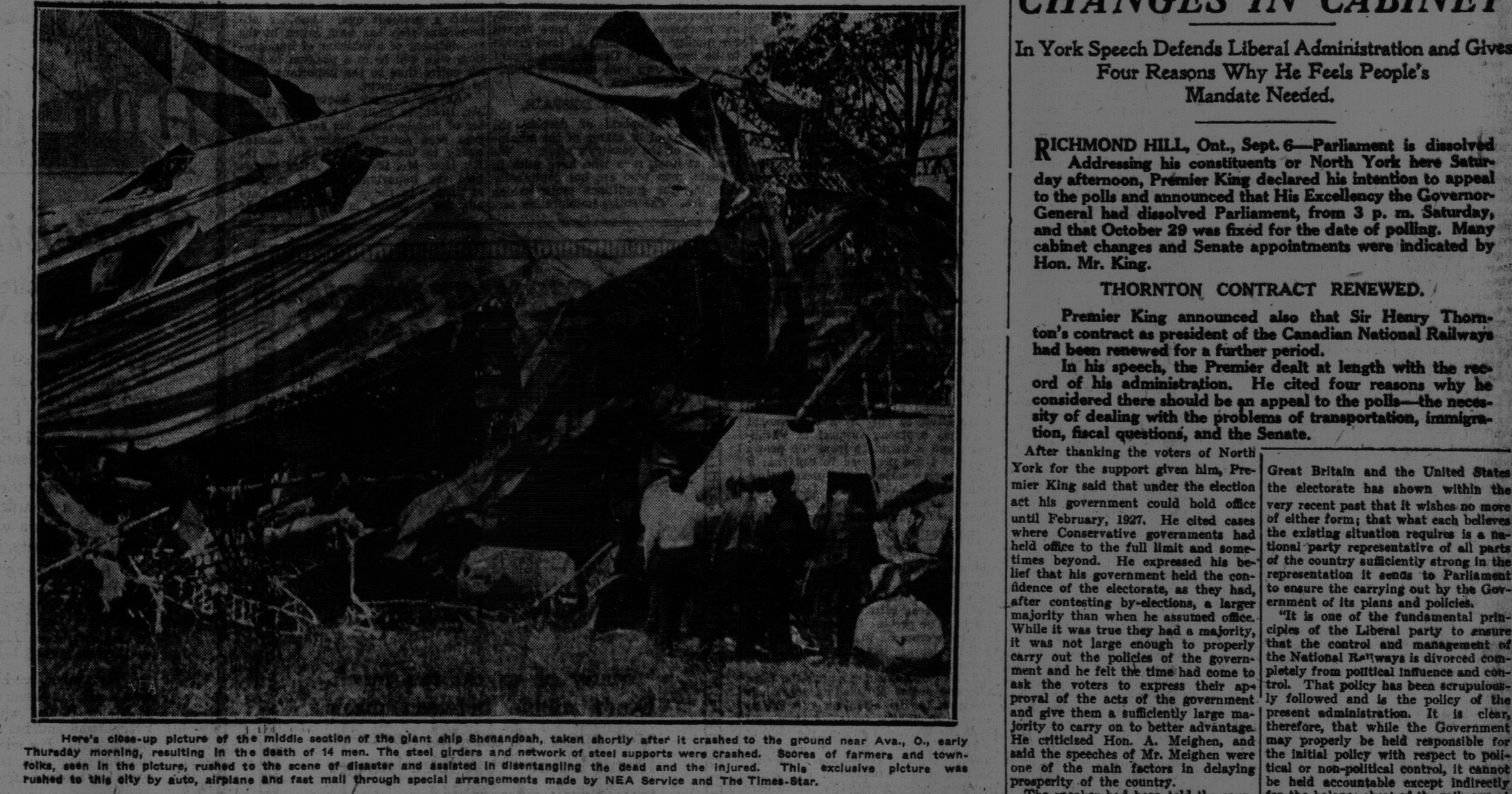
Here's close-up picture of the middle section of the giant ship Shenandoah, taken shortly after it crashed to the ground near Ava, O., early Thursday morning, resulting in the death of 14 men. The struts and network of steel supports were crushed. Scores of farmers and town-folks, seen in the picture, rushed to the scene of disaster and assisted in disintegrating the dead and the injured. This exclusive picture was taken to this city by auto, airplane and fast mail through special arrangements made by NEA Service and The Times-Star.
