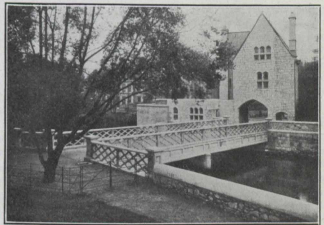
Fig. 1.—Reinforced Concrete Bridge.
