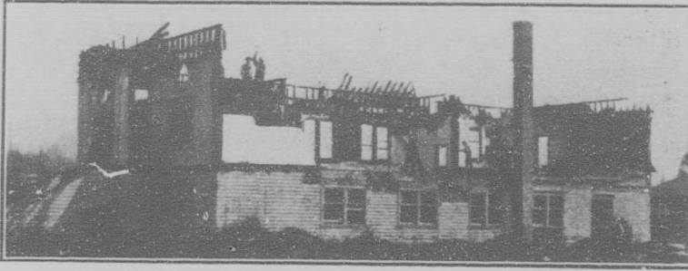
The Institute Hall After the Fire.
