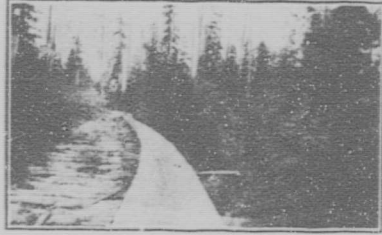
Continuation of Flume Past the Tennis Court near Mr. T. A. Allan's Residence.
