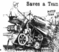
Cushman 4-Cycle Gasoline Engines have established their reputation for reliability under the hardest test ever given a farm engine—attached to the rear of a binder in the harvest field. Thousands are in use, doing all farm work, that were bought to use on binder. Fits any binder. Engine drives sickle and all machinery, leaving the horses nothing to do but pull the binder.
