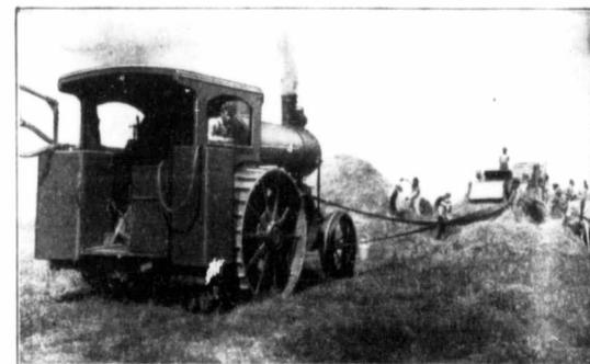
Avery Double Cylinder Undermounted Steam Engine. Three Sizes: 20, 30 or 40 H.P.
