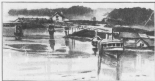
THE BRIDGE AND STEAMER "NORTHERN."
