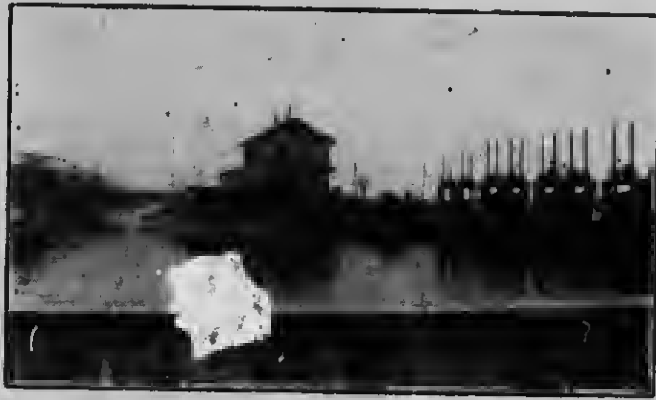
Fig. 1.—Vigevano, Forebay and Gates.
