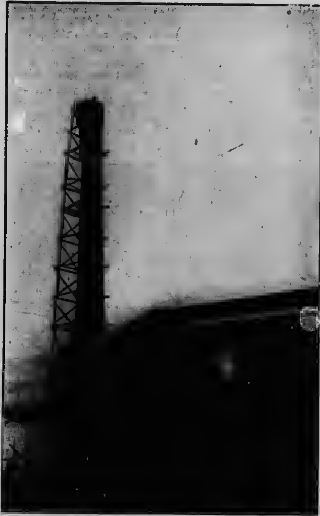
Fig. 5.—Terminal Overflow Pipe, Champ Station.
