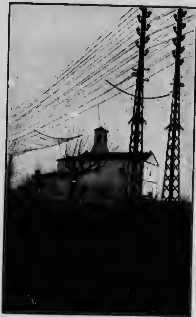
Fig. 4.—Paderno: Transmission Line, showing a Roadway Crossing.
