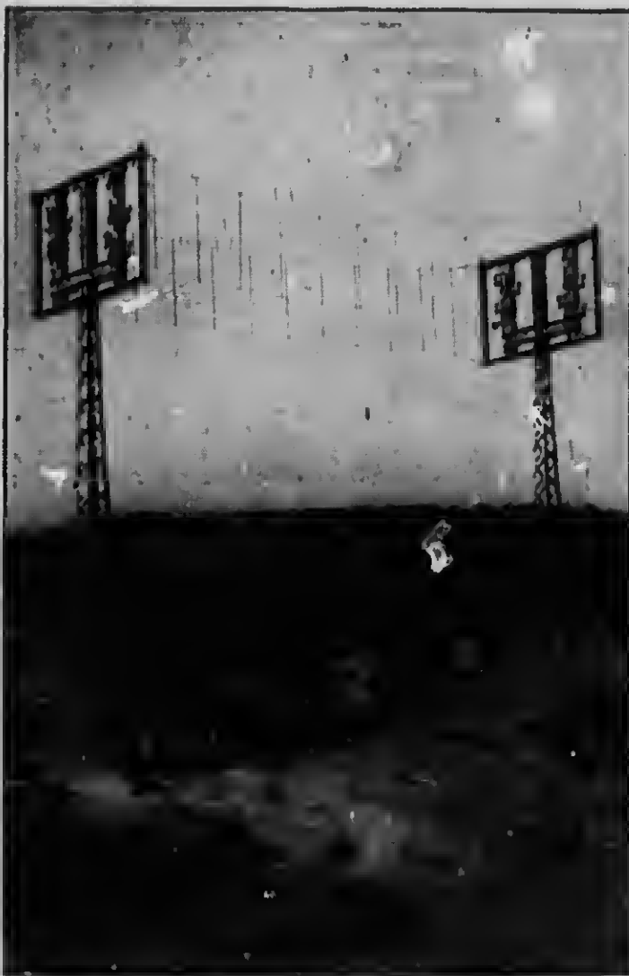
Transmission Line: Clermont-Ferrand, Railroad Crossing.
