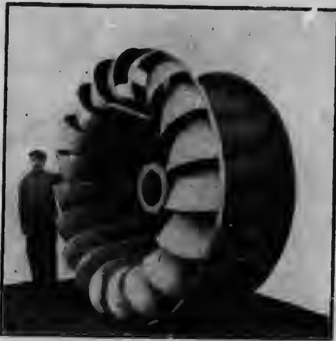
Fig. 10.—11'-0" diameter Runner for 9'-0" head.
