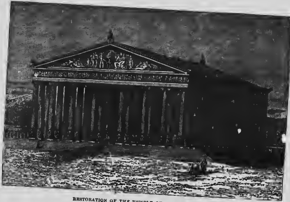
RESTORATION OF THE TEMPLE OF DIANA, EPHESUS. (By permission, from Wood's "Ephesus.")
