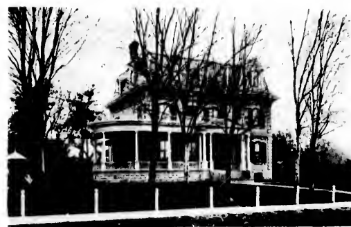
RESIDENCE OF GEORGE ROBINSON.
