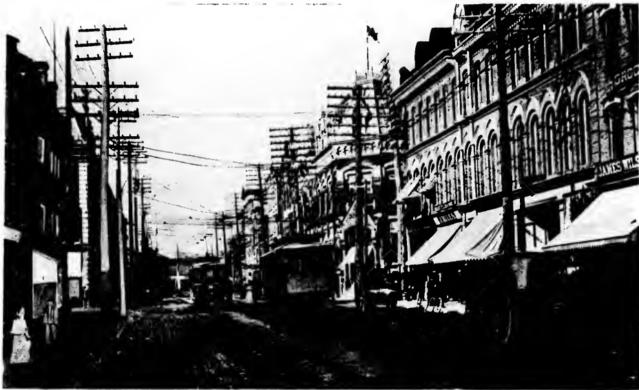
RICHMOND STREET, LOOKING NORTH FROM CITY HALL.
