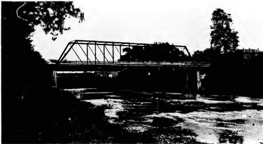
KING STREET BRIDGE, CARRYING TRUNK SEWER.
