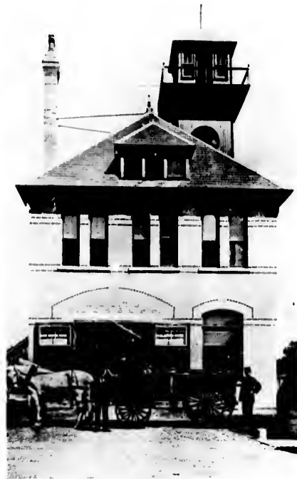
NO. 3 FIRE STATION.
