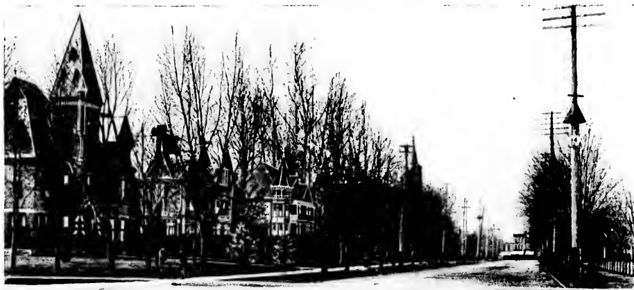
DUFFERIN AVENUE, SOUTH OF VICTORIA PARK, LOOKING WEST FROM WELLINGTON STREET.
