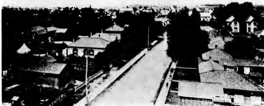
VIEW, LOOKING NORTH FROM EASTERN FIRE HALL NO. 2.
