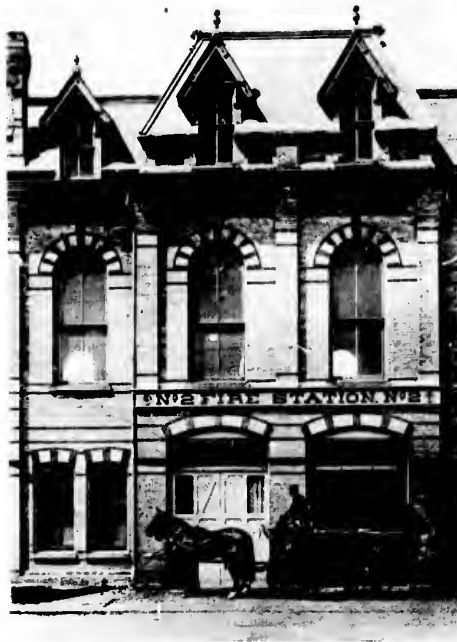
NO. 2 FIRE STATION.
