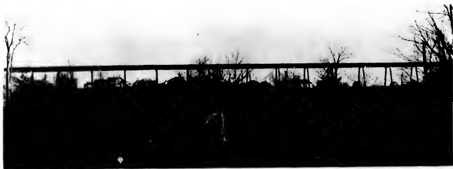
MILL CREEK BRIDGE, ON L. E. & D. R. RAILWAY — LENGTH 517 FEET 8 INCHES, HEIGHT 70 FEET.
