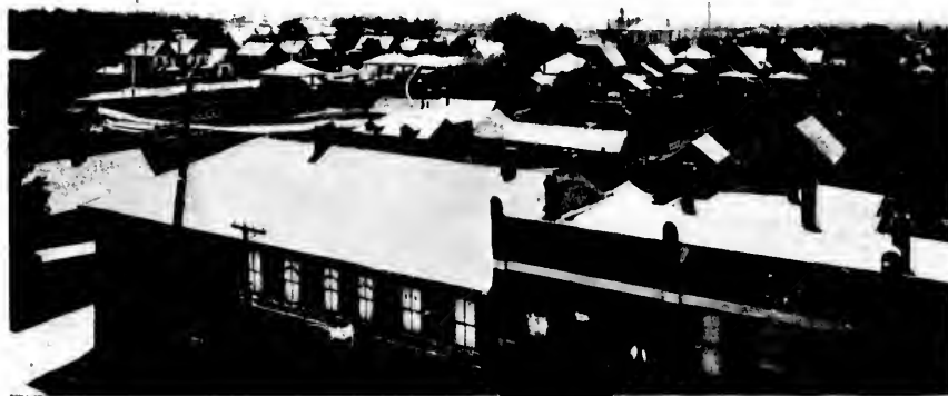
VIEW, LOOKING SOUTH-WEST FROM NO. 2 FIRE HALL.
