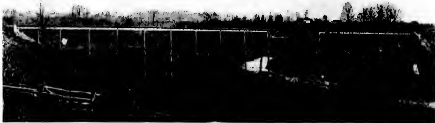
KETTLE CREEK BRIDGE, ON L. E. & D. R. RAILWAY — LENGTH 613 FEET, HEIGHT 73 FEET.
