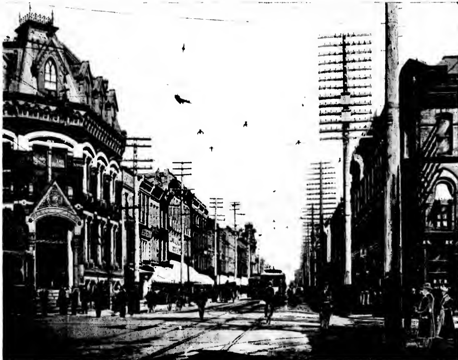
DUNDAS STREET, LOOKING EAST FROM RICHMOND.
