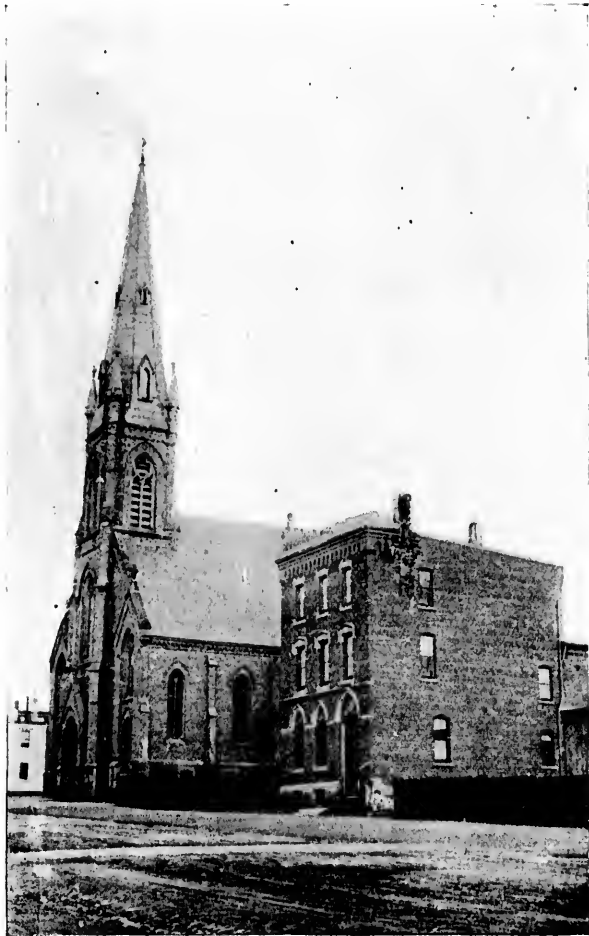
CHURCH OF ST. JOHN THE BAPTIST AND PAROCHIAL RESIDENCE, Broad Street, St. John, N. B.
