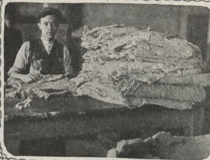
Extricating by the use of pincers any impurities remaining in crude rubber after it has been washed and oven-dried.
