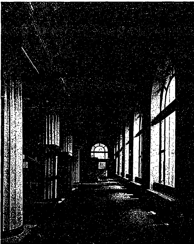
DETAIL OF BANKING ROOM.
