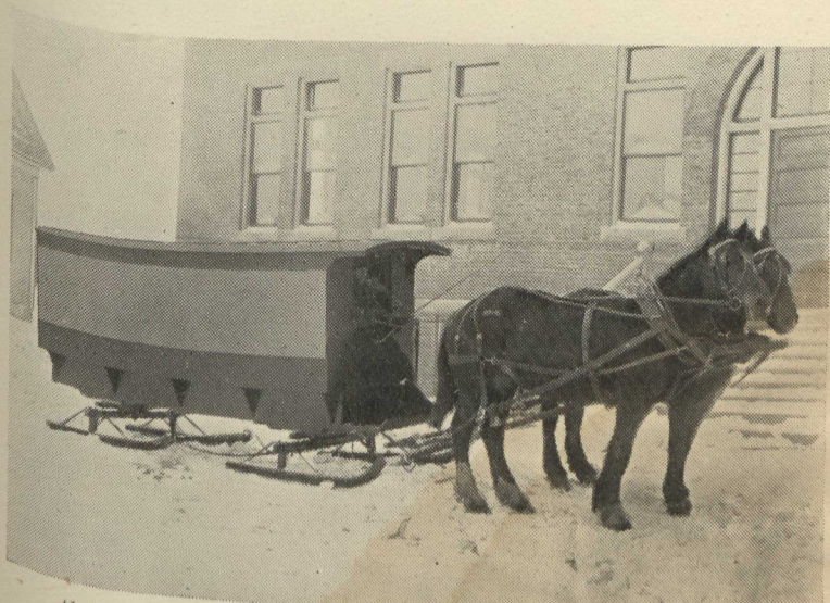
SCHOOL VAN (WINTER), MIDDLETON, NOVA SCOTIA. (Macdonald Consolidated School, 1904).
