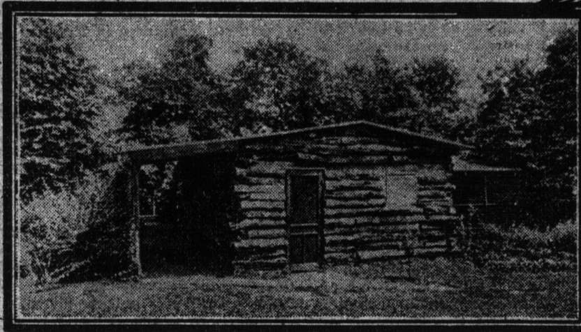
SEVEN HUNDRED OLD RAILWAY TIES TRANSFORMED INTO A BUNGALOW
