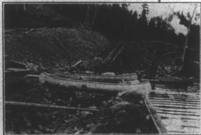
5000 tons of copper ore at the foot of Schist Lake. This will be hauled in winter to Sturgeon Landing, and then in summer to The Pas.
