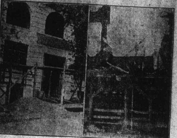
Shed in right picture saved lives at the new Equitable Building when a derrick and beam fell. It was built under strict supervision. The other shed was built at will.
