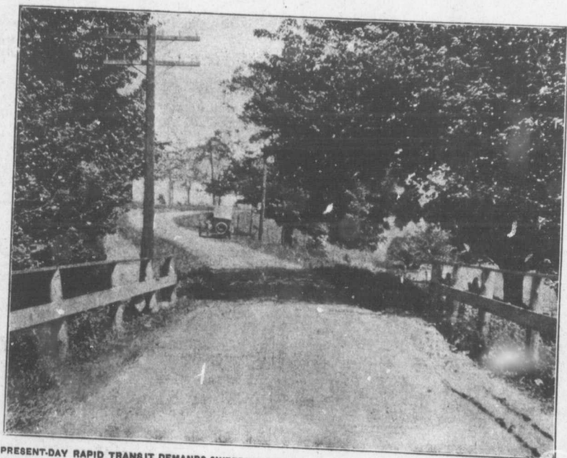
PRESENT-DAY RAPID TRANSIT DEMANDS SWEEPING CURVES AND CLEAR LOOKOUTS IF ACCIDENTS ARE TO BE AVOIDED.
