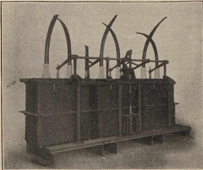
Type G Oil Circuit Breaker—Electrically Operated.
