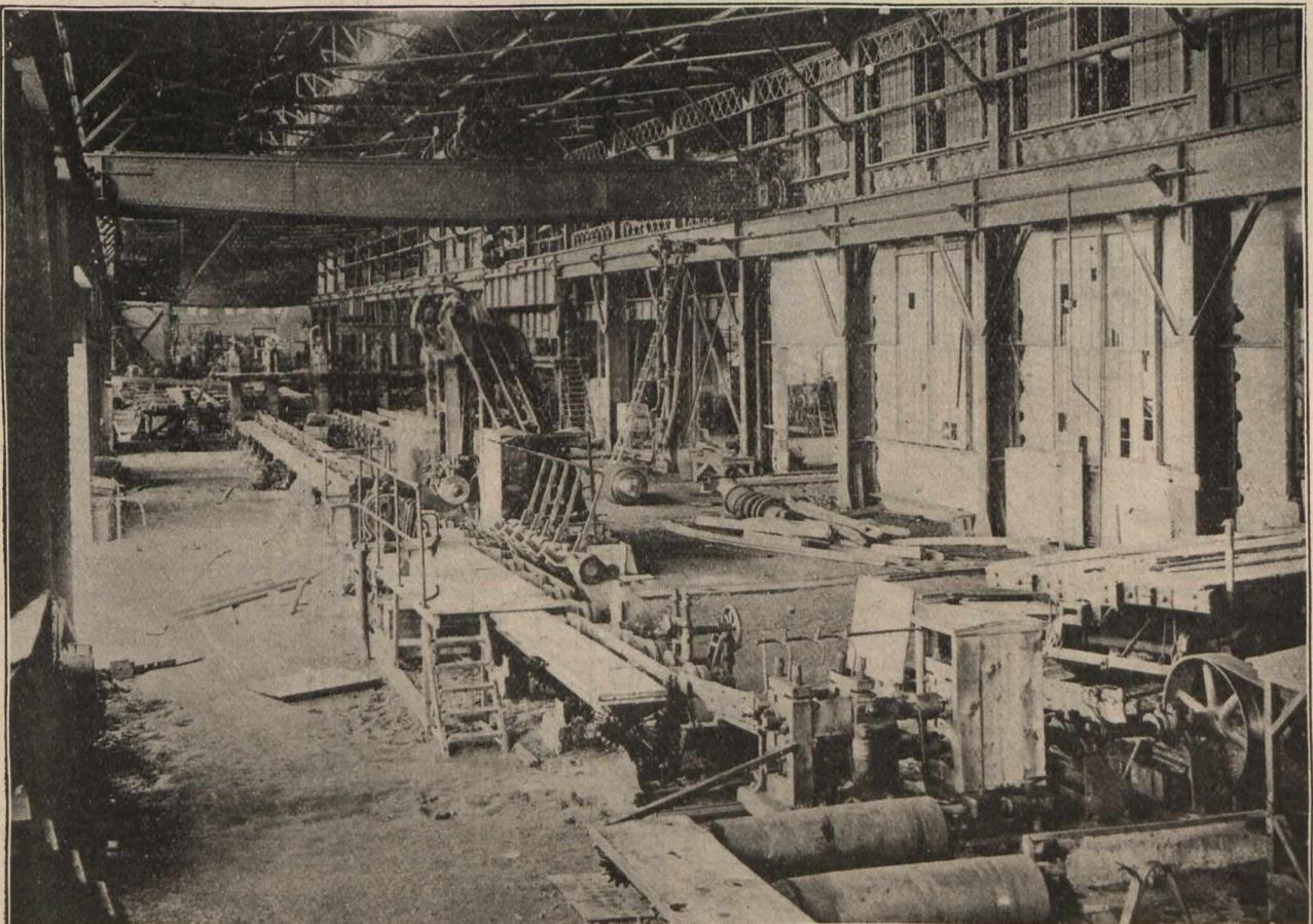
View of Back Side of the Mill Showing Cambering Machine, Stamping Machine, Rail Stops, Hot Saw and Tables.
