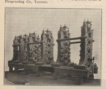
Roll Housings Assembled in Shop on Temporary Shoe Plates.
