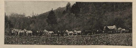
An 18-Horse Team Hauling the Lower Half of the Stator of an 750-k.w. Bullock Alternator Over 50 Miles of Mountain Road from the nearest Railroad Station to the Plant of the North Mountain Power Company.
