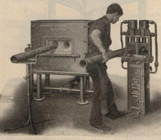
Fig. 2. Flue-Welding Furnace.
