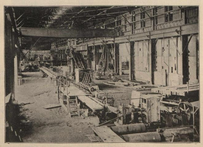
View of Back Side of the Mill Showing Cambering Machine, Stamping Machine, Rail Stops, Hot Saw and Tables.
