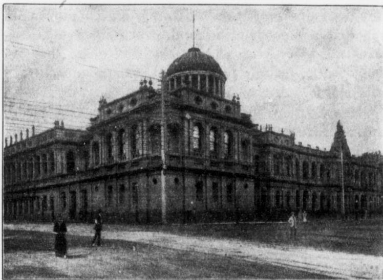
FIG. 31.—THE LAW COURTS, MELBOURNE. (Phot. C. Rudd, Melbourne.)
