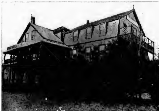
STRATTON HOUSE, FROM LAWN.
