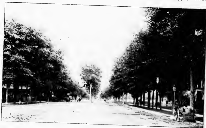
VIEW ON CIRCULAR STREET.
