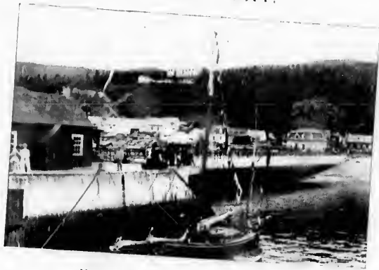
WHARF AT MURRAY BAY.
