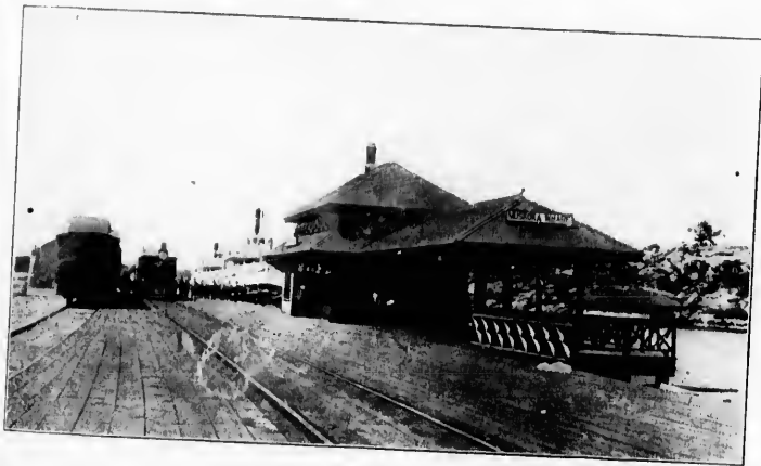
MUSKOKA WHARF STATION.
