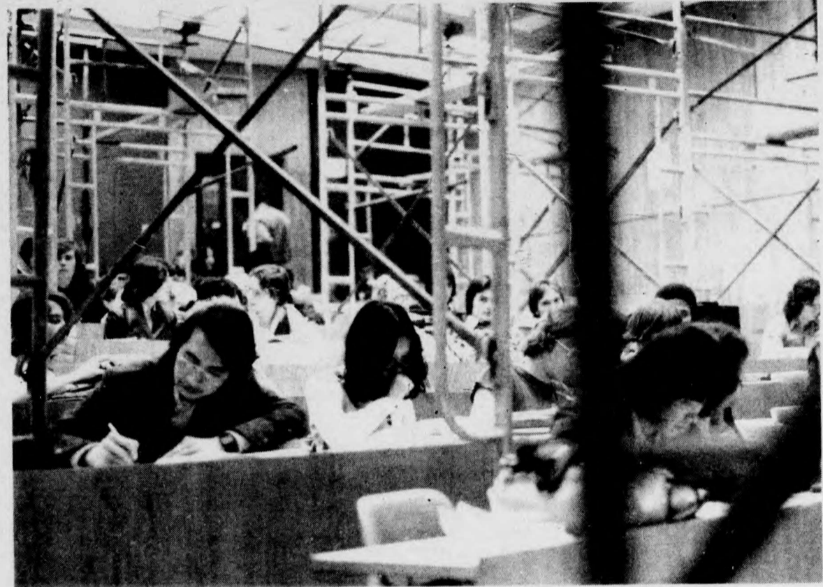
The collapse of Curtis lecture hall 110 made more than a few people wonder about York's stability. Steel supports now prop up a majority of lecture
