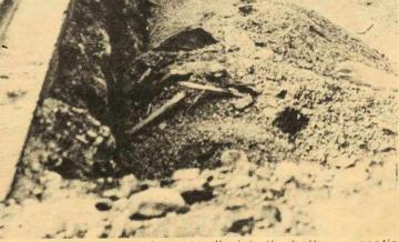
Is Dalhousie building a subway to alleviate the trattic congestion . the excavations on University Avenue on campus? Not quite . are for a heating duct to link the upper campus with the heating plant in the Tupper building.
