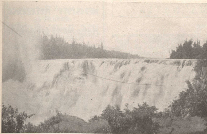
Power for the Twin Cities in Kakabeka Falls.
