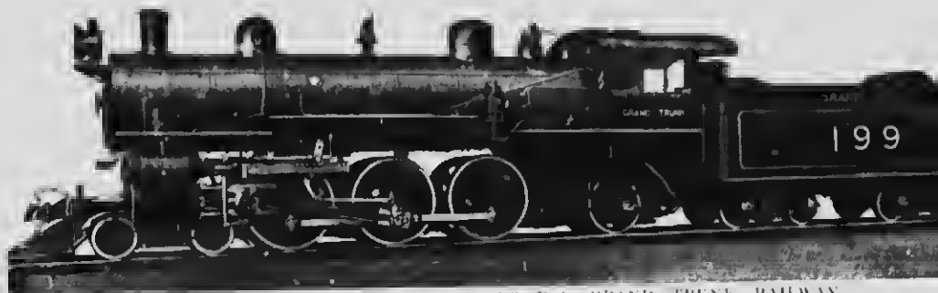
PACIFIC TYPE LOCOMOTIVE BUILT FOR GRAND TRUNK RAILWAY Total Weight of Engine, 226,000 pounds; Weight on Drivers, 115,500 pounds; Diameter of Drivers, 60 inches; Boiler Pressure, 185 pounds; Cylinders, 23 x 28 inches; Maximum Tractive Power, 33,900 pounds.
