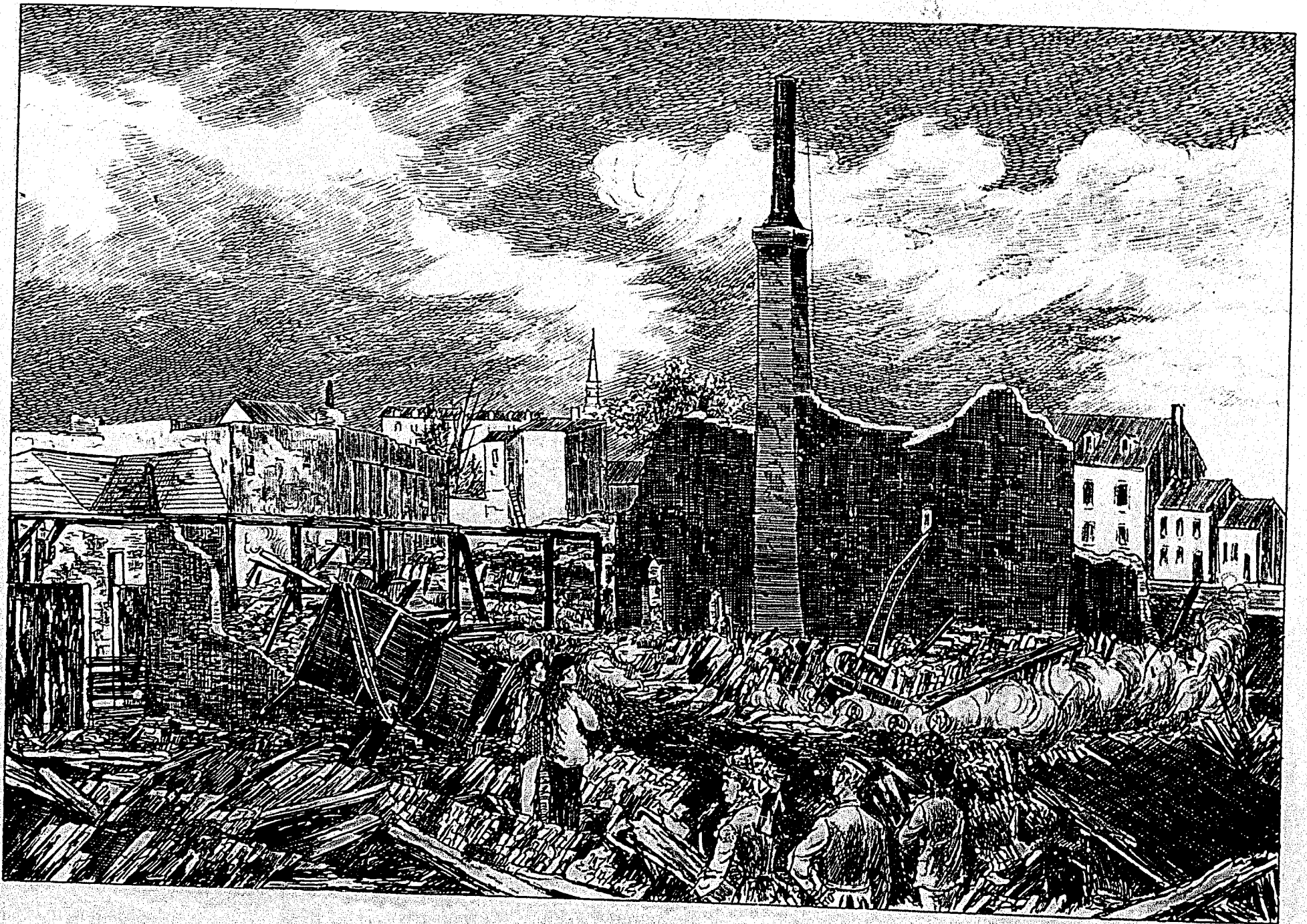
MONTREAL.—FIRE AT HOWLEY'S SASH AND DOOR FACTORY. VIEW OF THE RUINS.
