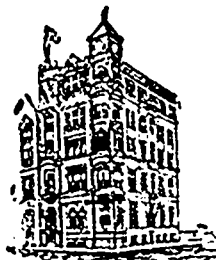
HEAD OFFICE BUILDING, MONTREAL.
