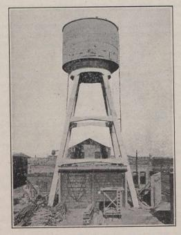
View Showing Elevated Concrete Tank.
