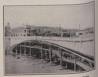
Fig. 7.—Testing Bridge by Seven Steam Rollers.
