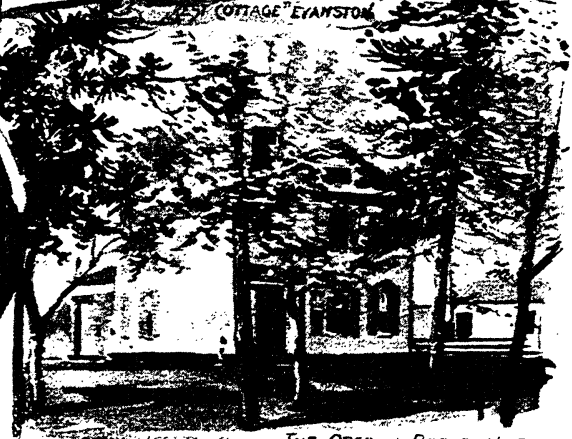
THE OBERLIN RESIDENCE
