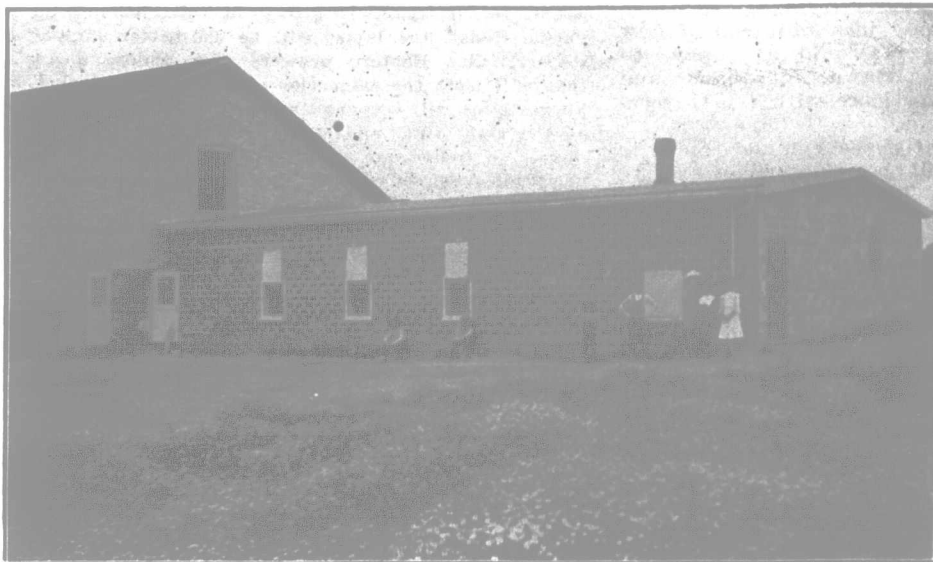
The Modern Cool-curing Room at the Harrietsville Cheese Factory.
