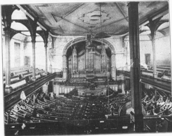
INTERIOR OF GRACE CHURCH, WINNIPEG.
