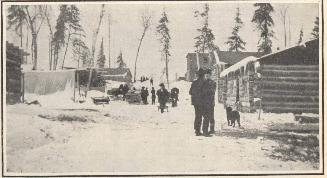
The New Silver Town in Northern Ontario.—Main Street in the Making.
