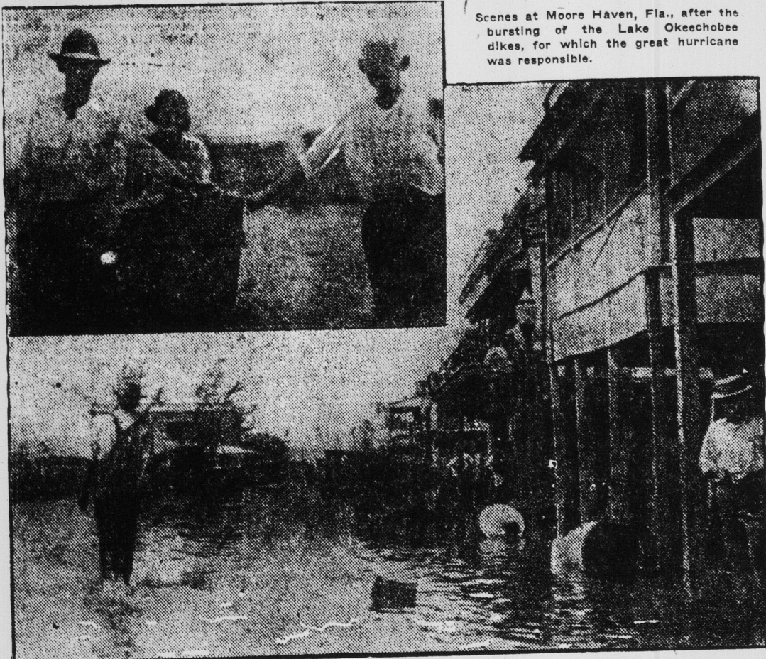
The Everglades city of Moore Haven, Fla., suffered far more from the floods which came with the breaking of the Lake Okechobee dam than from the Florida hurricane itself. Nearly a hundred persons are believed to have been drowned. Photos show Moore Haven's main street as the waters of the flood began to subside, making search for the dead possible; and a mother with her baby rescued in a small boat by two volunteer workers.
