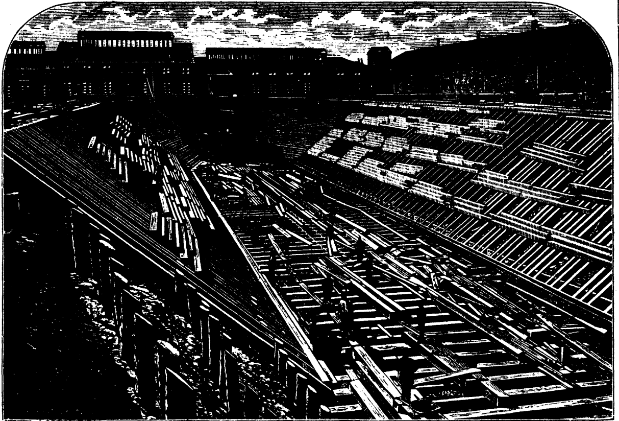
TIMBER DRY DOCK AT BALTIMORE, MARYLAND, U.S.A.
