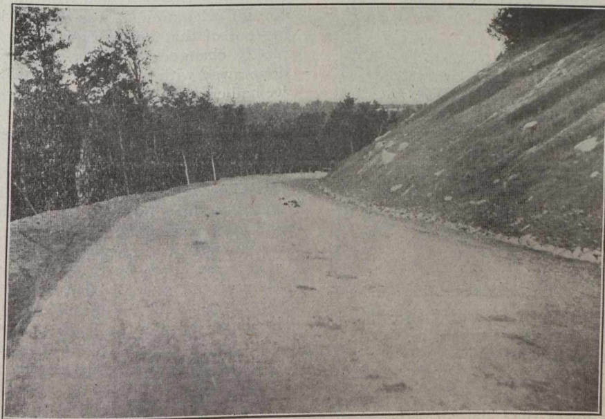
Fig. 1.—Montreal-Quebec Road, Donnacona (Portneuf). Macadam Done in 1915.
