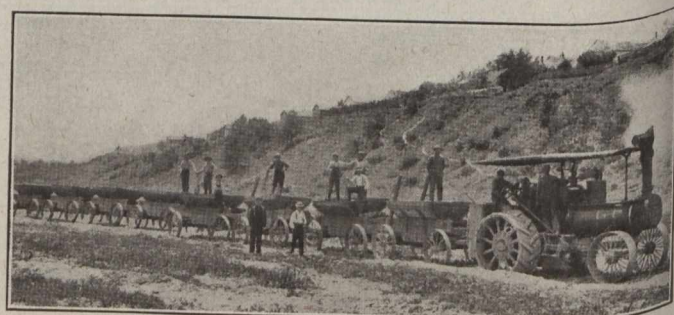
Fig. 4.—Levis-Jackman Road—St. Georges (Beauce). Conveying Gravel with a Traction Engine and Trucks.
