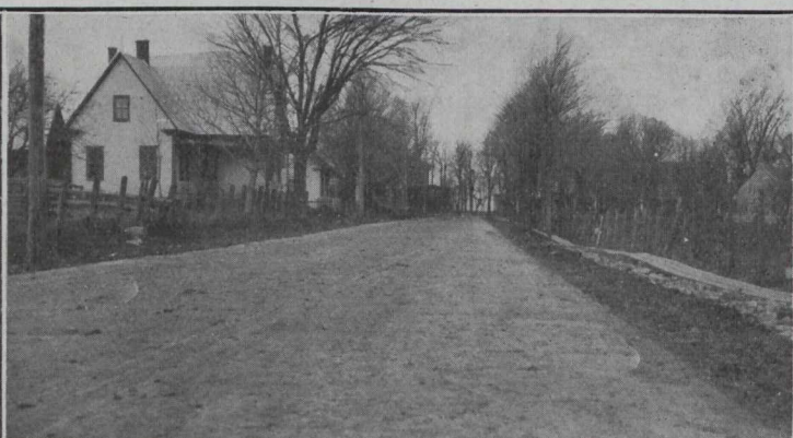
The Road Completed.
