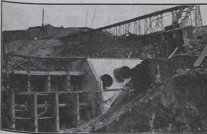
Down-Stream View of Dam, Showing Position of Steel Penstock.
