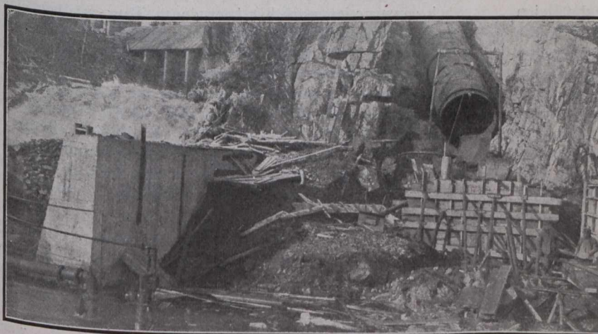
Eight-foot Steel Penstock from Power House Site.
