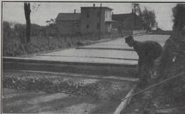
Crowning Road with Template, Napierville, Quebec.
