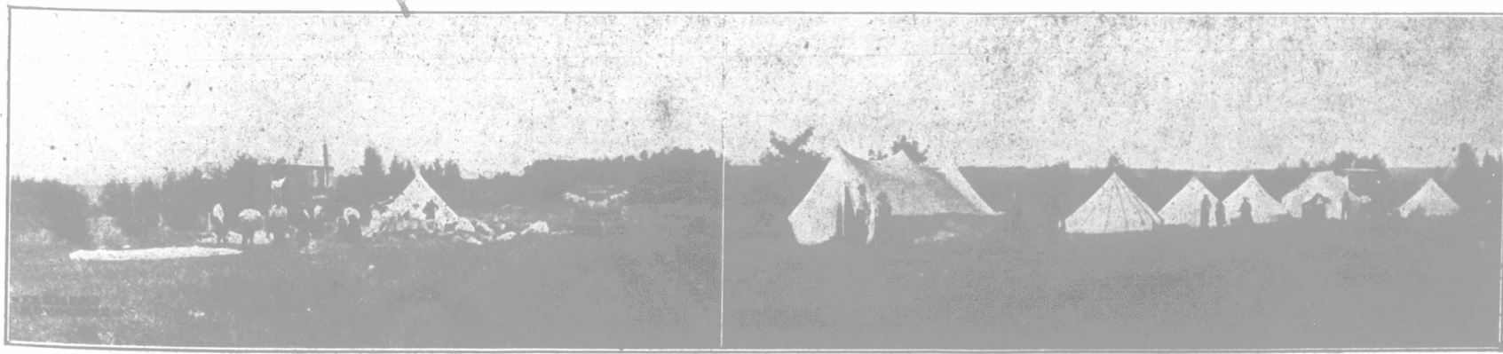
EQUIPMENT AND TENTS OF THOSE WHO BUILD TELEPHONE LINES. Gangs of men are at work in many parts of the West putting up rural telephone lines. A representative of the Farmer's Advocate took photographs near Franklin, Man. One shows the gang on arrival at a new tenting place and the other with tents pitched a short time after arrival.
