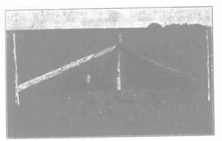
Proper Method of Bracing Corner Posts. In addition to these braces, the post should be thoroughly anchored at the bottom, especially where woven wire is used, as the strain on a corner post is heavy.
