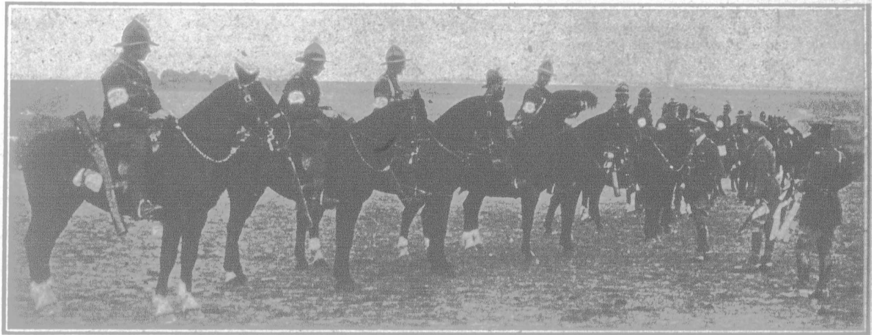
A New Zealand Division Horse Show on the Western Front.
